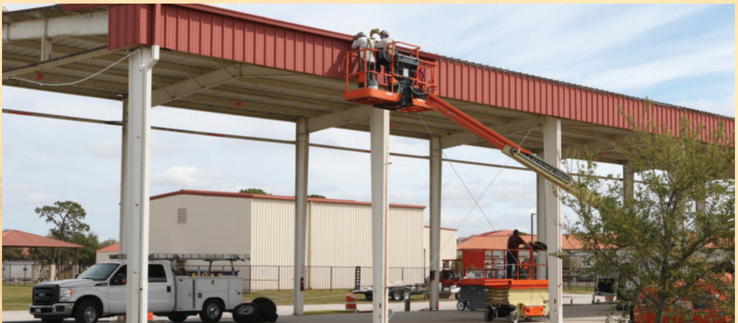
Construction workers began tear down procedures of the existing base supply and equipment shed, March 6, 2020, that has transformed into the new U.S. Special Operations Command-Central's human performance outdoor facility at MacDill Air Force Base, Tampa, Fla. Photo by U.S. Army Staff Sgt. Steven M. Colvin.
